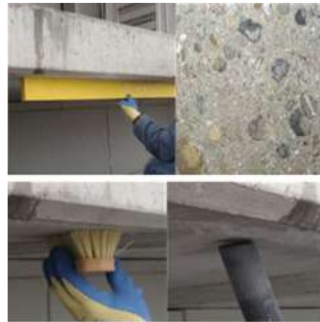
Figure 5 Surface leveling, and cleaning
