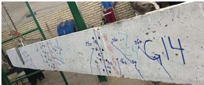
Figure 12 The patterns crack of beam G14.
