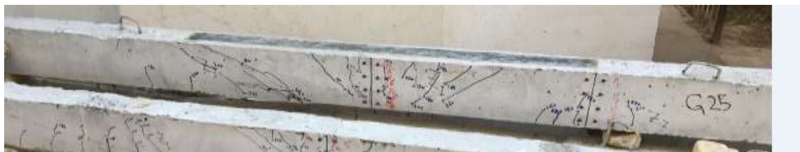
Figure 18 The patterns crack of beam G25.
