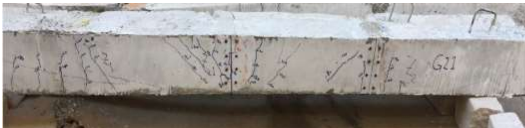
Figure 14 The patterns crack of beam G21.
