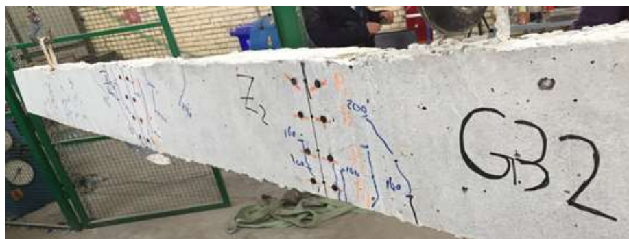
Figure 20 The patterns crack of beam G32.
