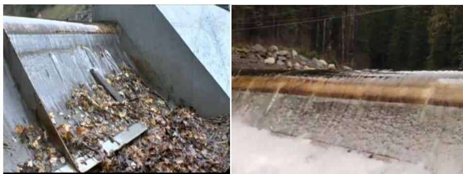
**Figure 1** Screen condition of tyrol weir which is sediment
