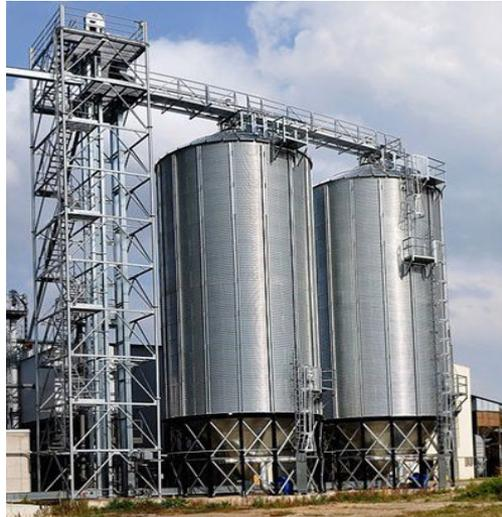
**Figure 4** Example of stiffened corrugated steel with conical hopper [17]
