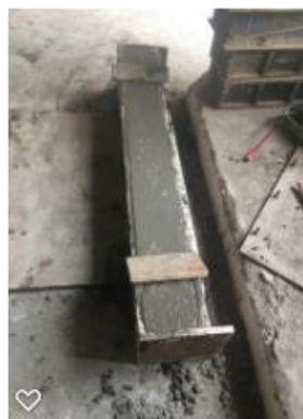
Figure 3 Final form of column cast
