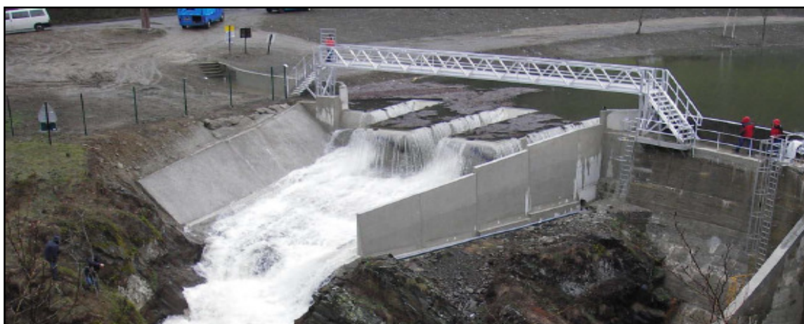
Fig. 2 Goulours dam, France with a Piano Key Weir
